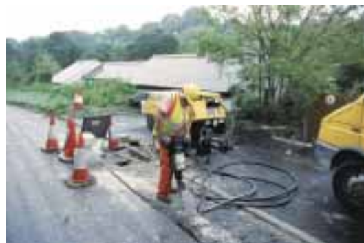
Use of a vibrating tool for road breaking
